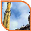
Flue Gas Scrubbing
